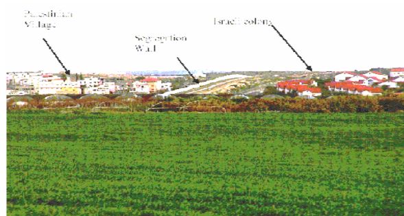
pic.5- Explaining the expansion and annexation wall near the settlements in the palestinian territories in qalqilia governorate.
