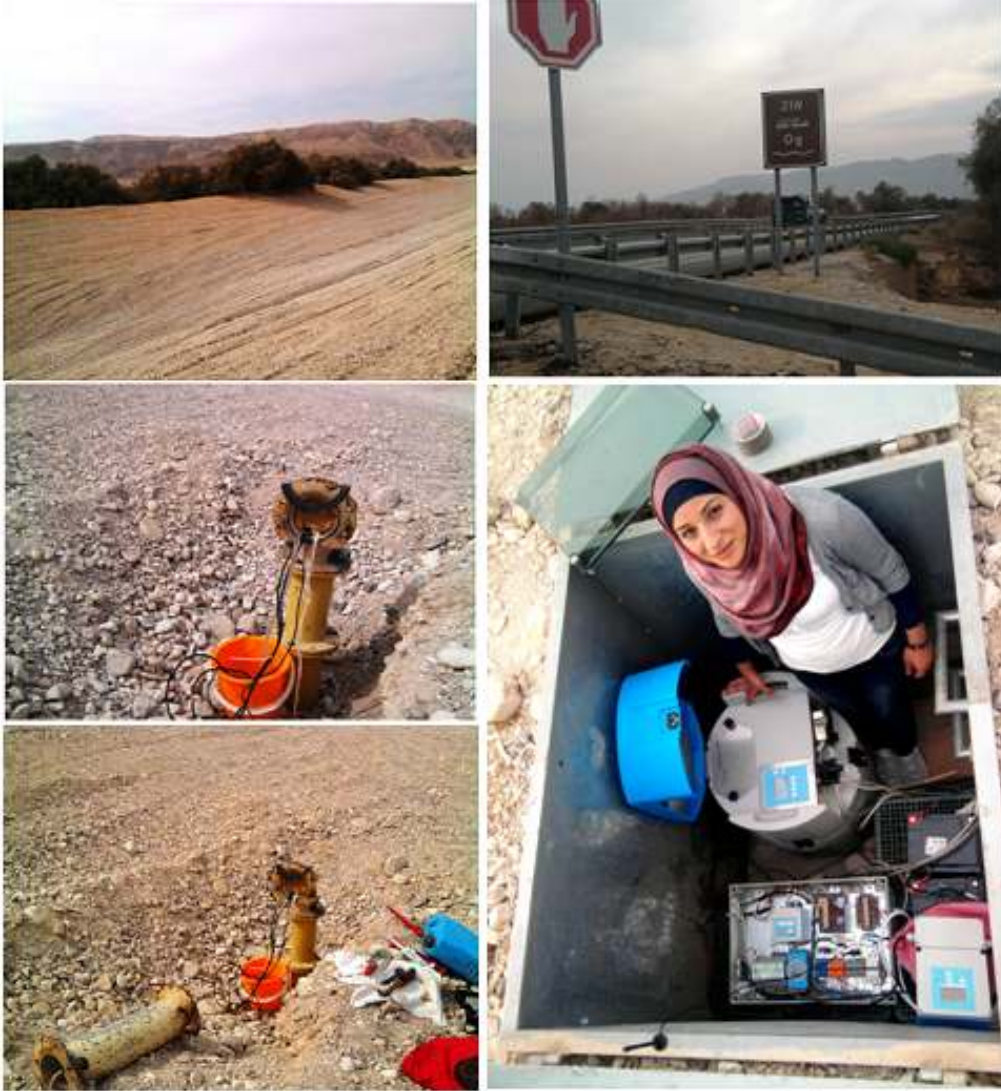
Figure (3-11): Testing the Og Hydrometric Station Prior Rainy Season
