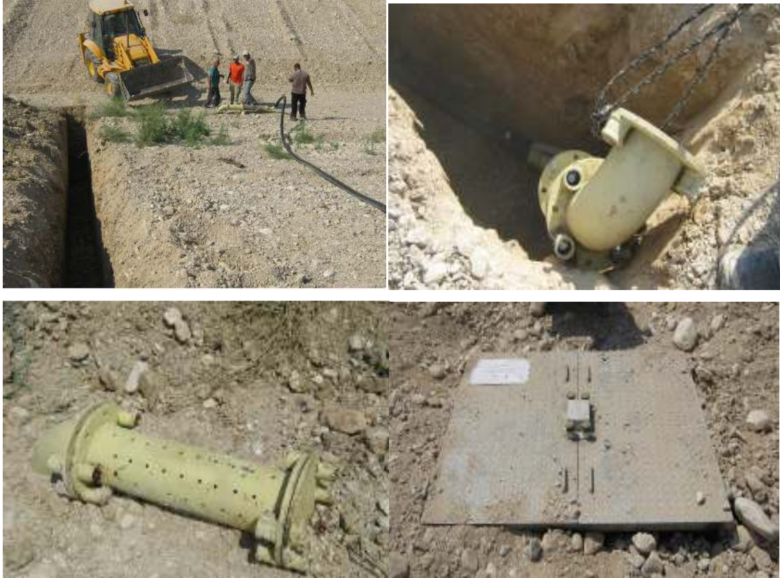
Figure (3-8): Perforated Pipe and Hydraulic Station Installation
